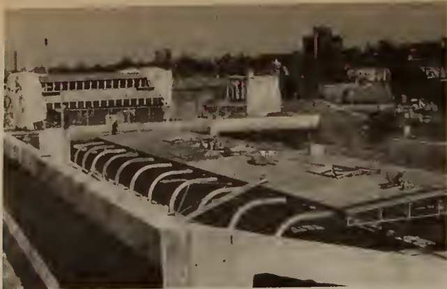
Green Street Station canopy roof near Gordon Street in Jamaica Plain.
